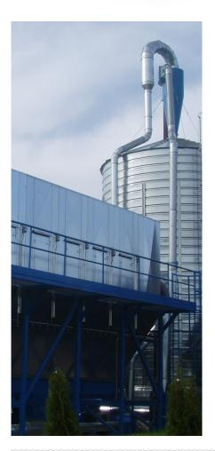
Recirculation filters, aspiration pipelines, fans and silos for wood processing enterprises and by-products processing mills.
